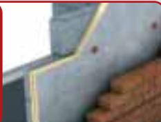
A photograph showing a cross-section of a building's exterior wall. It features a thicker, rigid insulation board (Polyiso Plus) applied over a metal cladding. The insulation board is shown in a corner joint, demonstrating its ability to fit into tight spaces.
