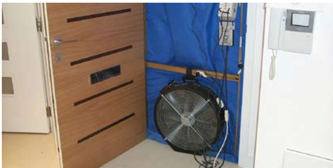
Figure 22 Fan pressurisation equipment used for dwellings
