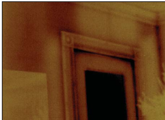
Image 4: Properly installed cellulose provides excellent insulation. However, quality problems can occur due to poor installation (with missed areas) and due to settling over time.
